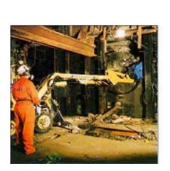
You improve the operators' working environment when the Brokk 250 is used for different kinds of building demolition. You spare operators the vibrations connected with the use of hand-held tools. And they can remain at a safe distance from falling debris, dust, and splinters.
